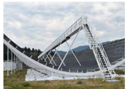
CHIME is a collaboration between the University of Toronto, University of British Columbia, McGill University, and Canada's Dominion Radio Astrophysical Observatory. Originally conceived to map the most abundant element in the universe, hydrogen, this unusual telescope has no moving parts and is composed of four large cylinders, 100 meters long and 20 meters wide each, arranged north-south, with a thousand detectors spread across them. CREDIT: Wikimedia Commons
